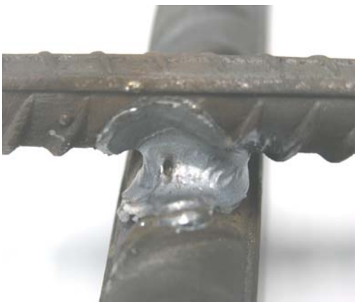
Figure 8. Example of Unacceptable Tack Weld Evidence of porosity & unacceptable undercut
